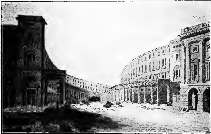
The Quadrant Colonnade in process of Construction. (From a unique picture by Charles Wild, in possession of Mr. James Tregaskis, dated 1812).
